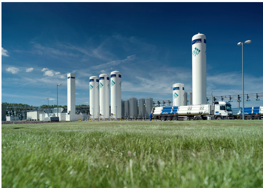
Figure 2. As thin film silicon fabs grow in scale, the economics favor on-site generation of major bulk gases such as hydrogen and nitrogen.
